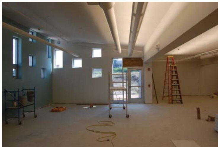
dorm area under construction
